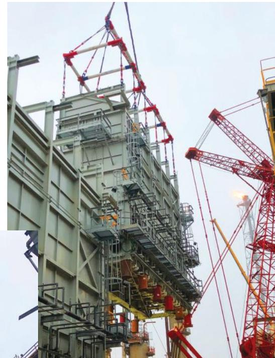
Successful 12-point super-lift ready for placement and fit up.
